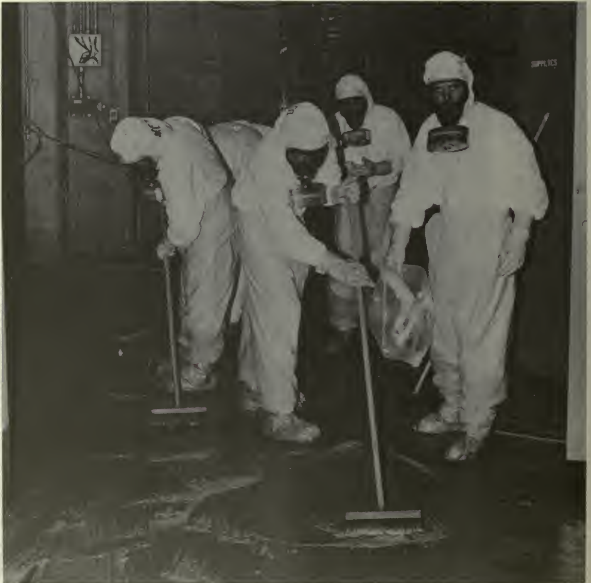
TMI personnel cleaning up the contaminated auxiliary building.
